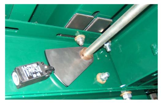
Here is how the new safety gear plate looks fitted on the inner part under the floor.
